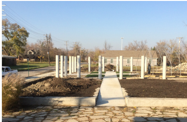
The Tunnel House and Market Plaza from Farmhouse Terrace looking towards the Art House
