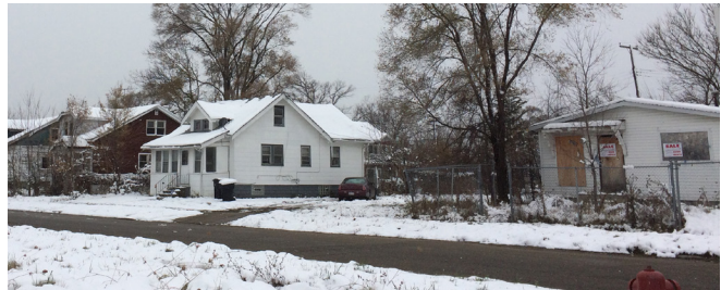
Typical existing neighborhood housing
