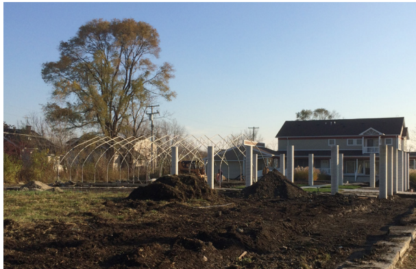
Looking across production bed area to Farmhouse—fencing to be installed
