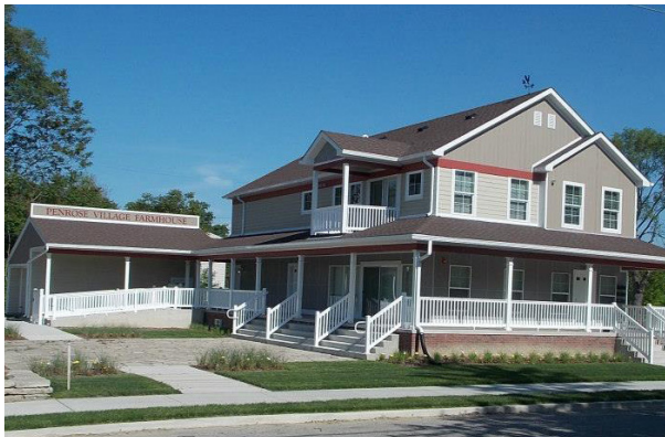
The Penrose Farmhouse on Charleston Street
