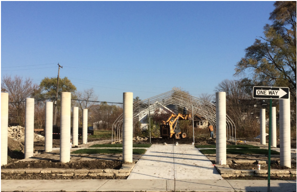
The Tunnel House and Market Plaza under construction
